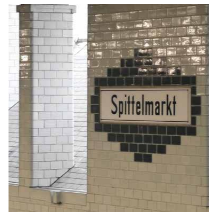
Underground station Berlin Spittelmarkt Replications of tiles in highest quality ensure a professional and renewal true to the original style and historic structure.
